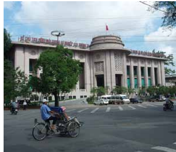
The headquarters of Vietnam's central bank in Hanoi. The central bank now holds a majority share in Ocean Bank, following its takeover of the troubled bank in April. https://www.flickr.com/photos/79893993@N00/2096886217
