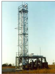
Pilot Plant Coweta Fixed Bed, 2 BPD
