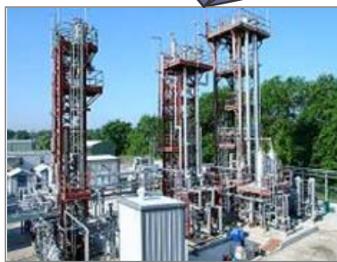
Tulsa Pilot Plant Fixed Bed, 2 BPD
