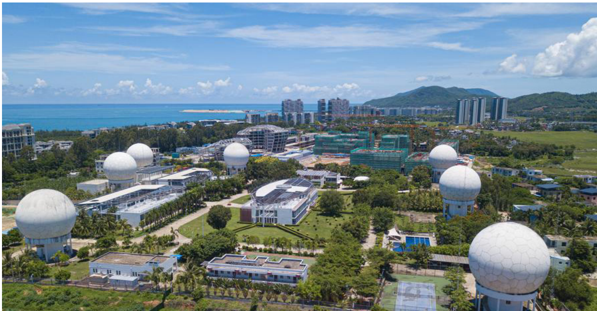
Figure 12: Aerial Photo of China Remote Sensing Satellite Ground Station at Sanya Remote Sensing Industrial Park on Hainan Island, July 5, 2024
