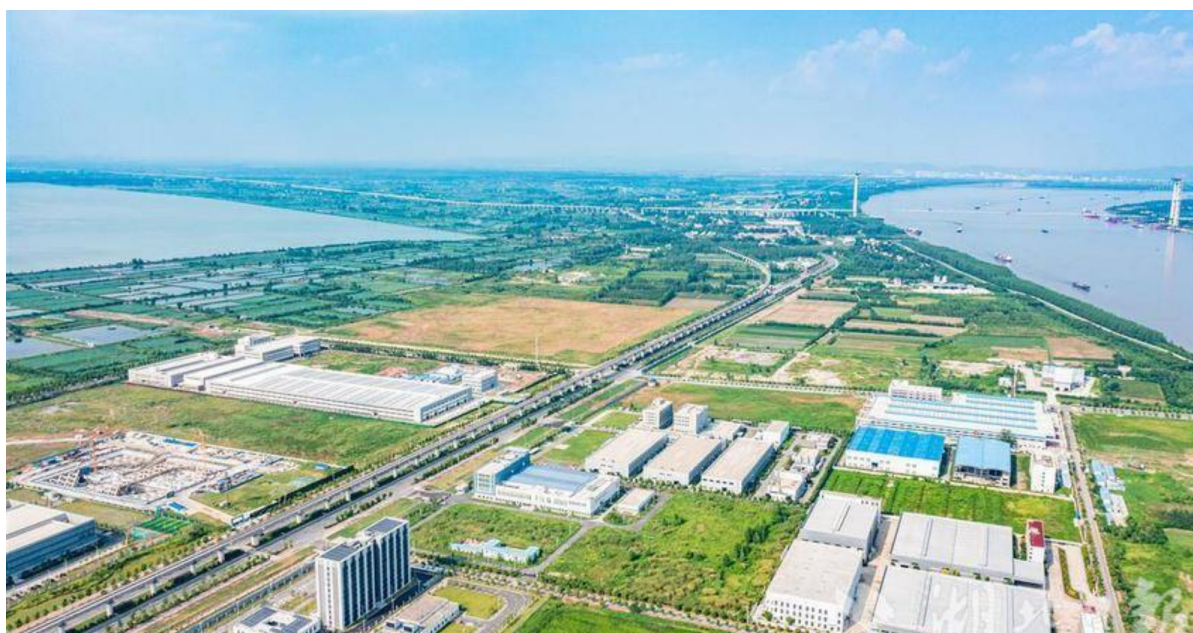
Figure 8: Aerial Photo of Wuhan National Aerospace Industry Base Under Construction, July 2025
