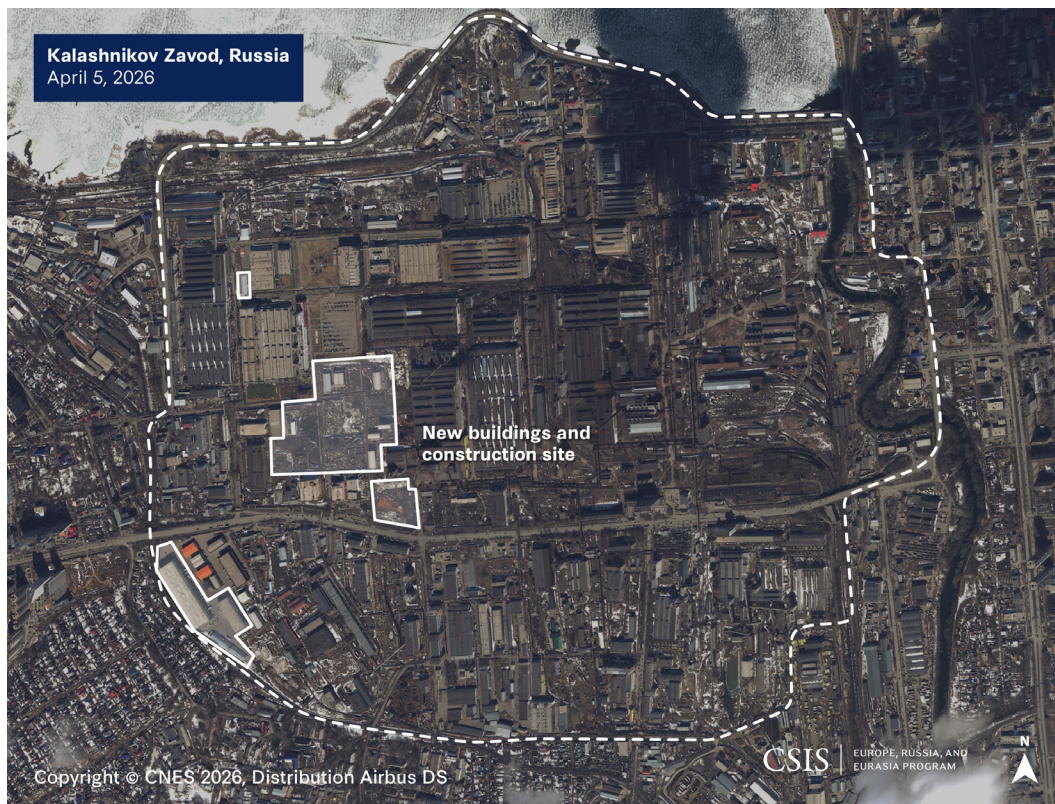
Figure 2a: Infrastructure Developments at Kalashnikov Zavod, 2026
