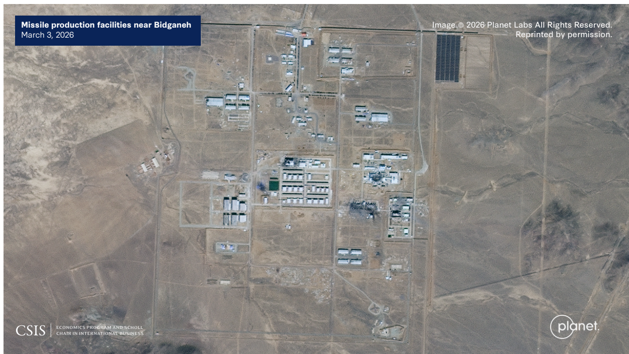
Figure 4: Damage to Missile Production Facilities near Bidganeh on March 3, 2026
