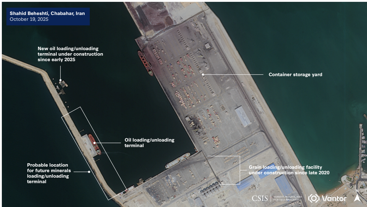
Figure 5b: New Oil Loading and Unloading Terminal, Shahid Beheshti Port, Under Construction in 2025
