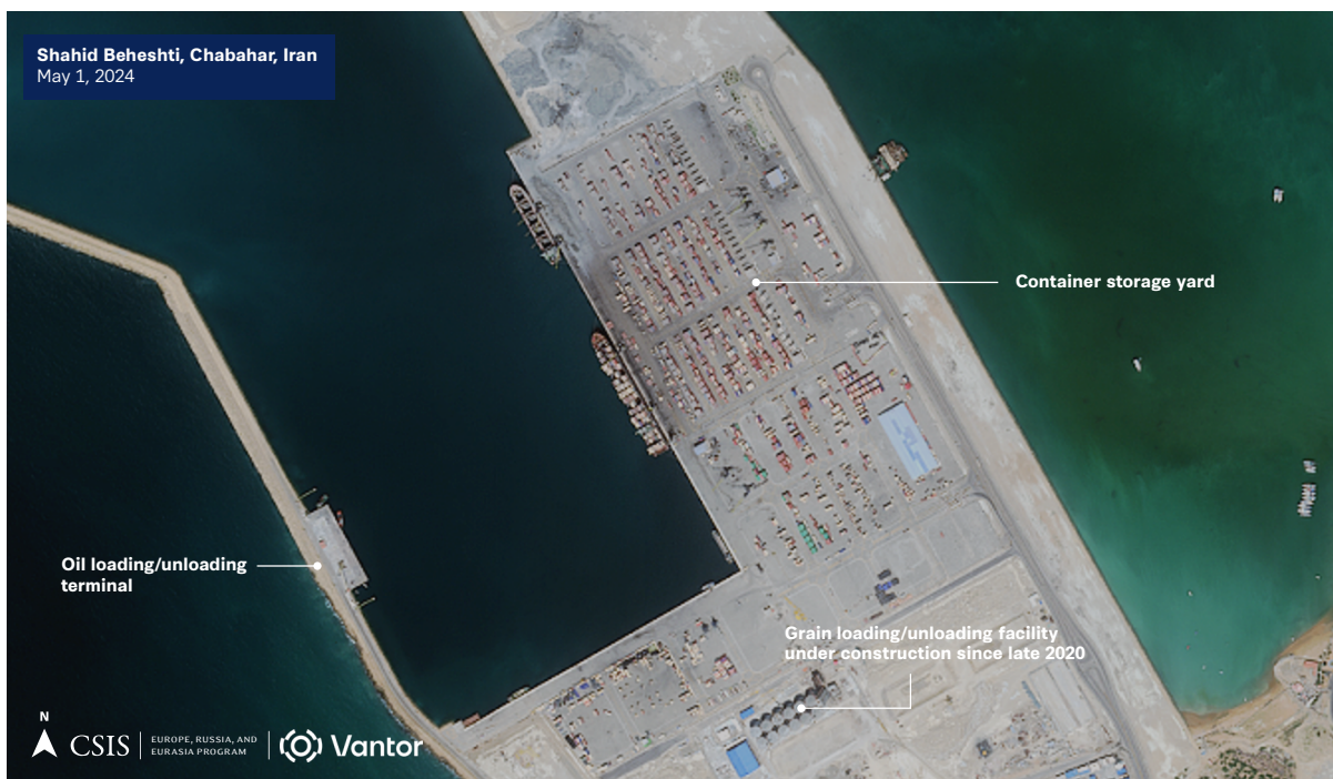
Figure 5a: Site of New Oil Loading and Unloading Terminal, Shahid Beheshti Port, 2024
