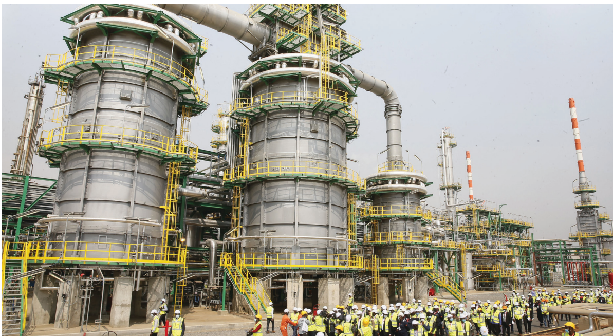
A general view of the refinery at the state oil company, Sonangol, in Luanda, Angola, on June 7, 2022.
